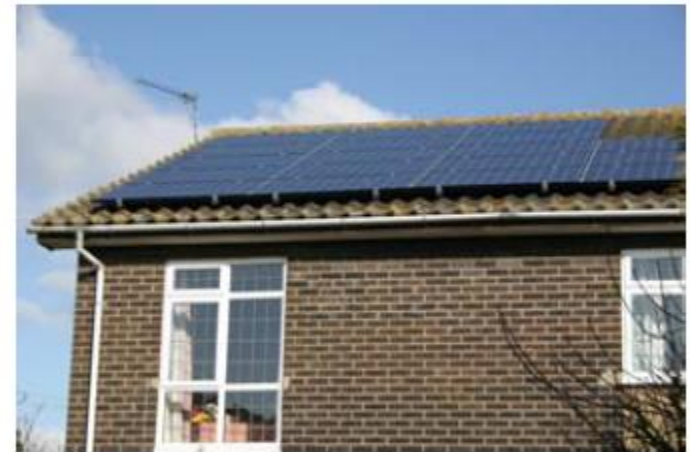
Figure 6.5. Solar photovoltaics: data from a 25-m 2 array in Cambridgeshire in 2006. The peak power delivered by this array is about 4 kW. The average, year-round, is 12 kWh per day. That's 20 W per square metre of panel.
