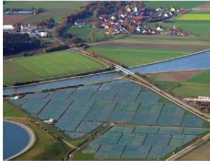
Figure 6.7. A solar photovoltaic farm: the 6.3 MW (peak) Solarpark in Mühlhausen, Bavaria. Its average power per unit land area is expected to be about 5 \text{ W/m}^2 . Photo by SunPower.
